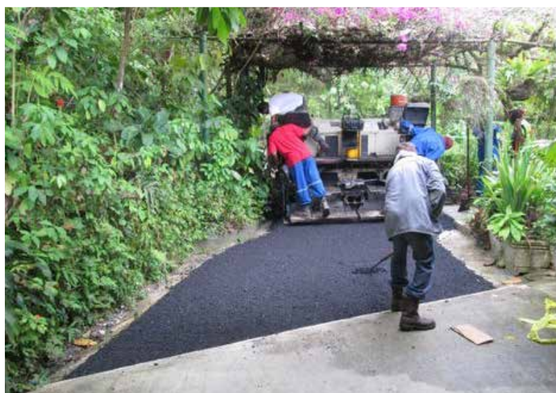
From the doorstep to the main road
